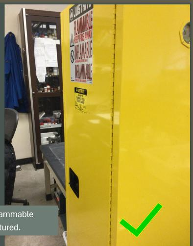
Flammable storage cabinets have working self-closing doors and otherwise meet Calif. fire code and Cal/OSHA regs
